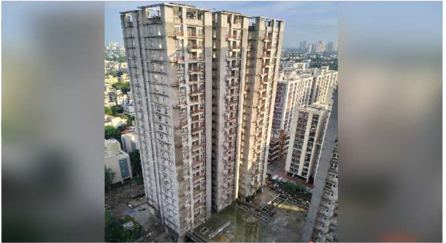
BLOCK - 3 EXTERNAL VIEW
